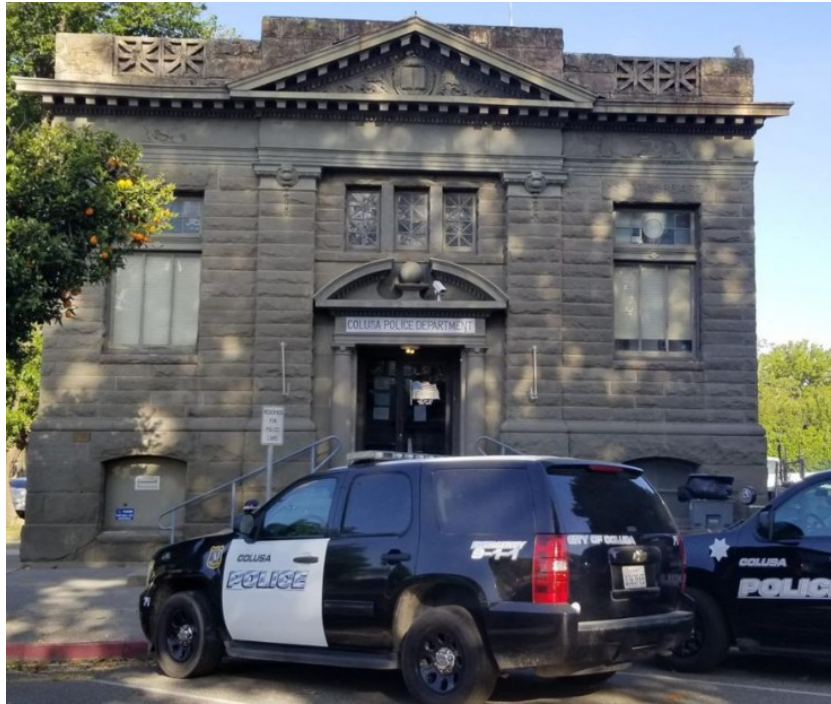
Existing Police Station at 206 6 th Street
