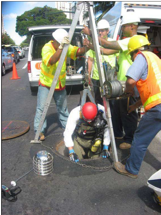
Photo 3.1 – Confined Space Entry
